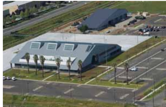
The Sacramento Readiness Center (foreground) and Field Maintenance Shop, located on Okinawa Street at the former Sacramento Army Depot
