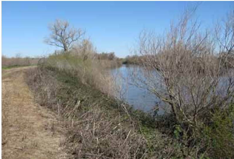
Waterside condition in area to be degraded (will be cut down approximately 9 feet)
