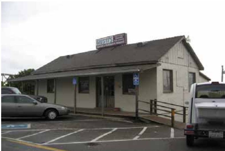
Upgrade to PL 84-99 not possible due to presence of the structure on top of the levee
