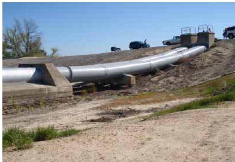
Northeastern landside view of EBMUD aqueduct penetration into the levee
