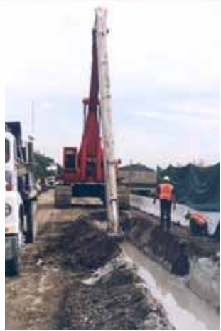
Seepage remediation by cutoff wall
