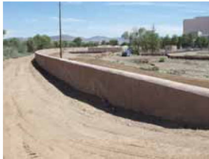
Reno-Sparks Indian Colony Floodwall
