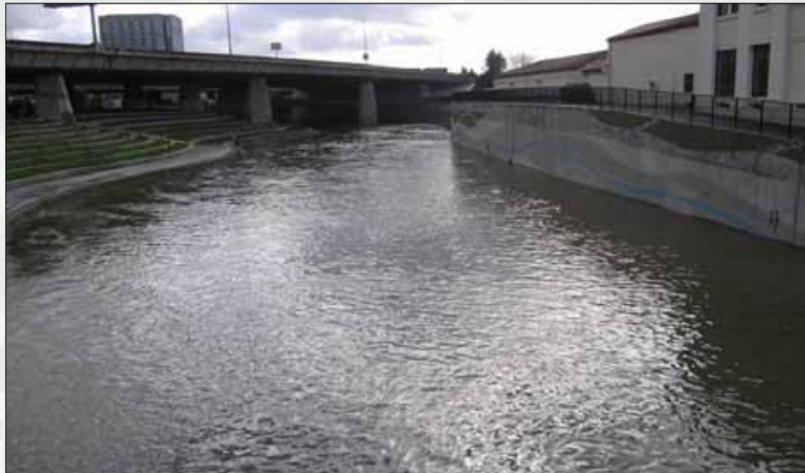
Contract 3B: Santa Clara Street Looking Upstream
