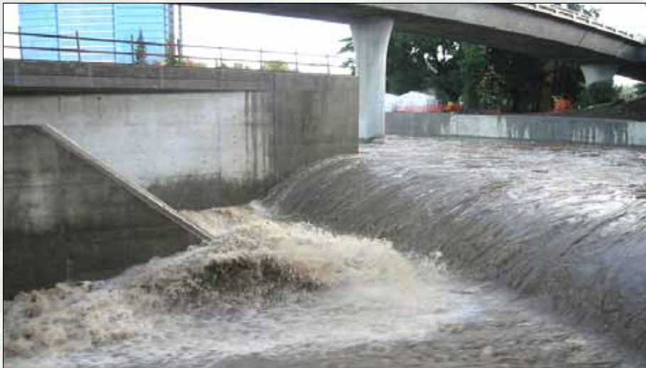
Contract 3C: Woz Way Bypass Inlet (Winter 2002)
