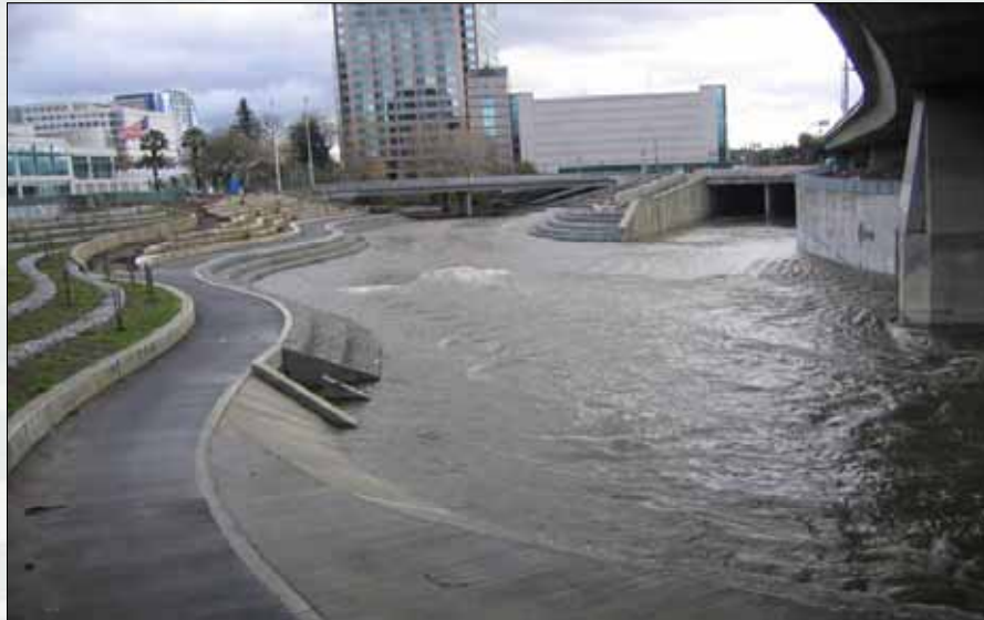
Contract 3B: San Fernando St. looking U/S (Bypass Outlet)
