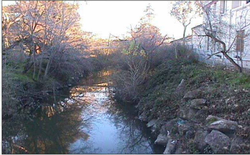
Contract 3B: Santa Clara Street Looking Upstream (Pre-project)
