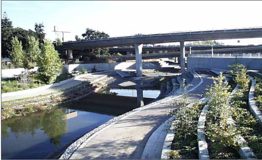
Contract 3C: Woz Way looking upstream
