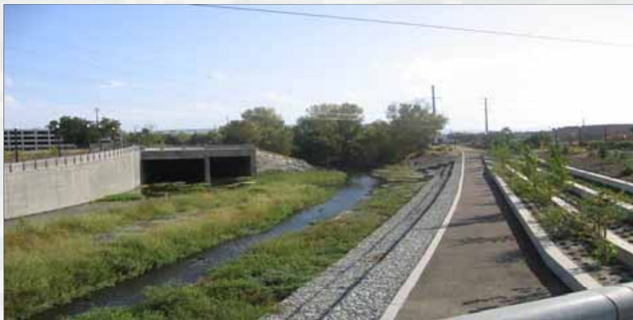
Contract 3A: Coleman Avenue Looking U/S (Bypass Outlet)
