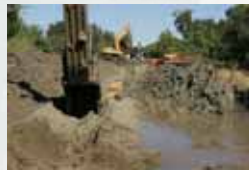
Slurry Wall Construction
